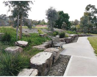
figure 5 Stone retaining wall and planted embankment
